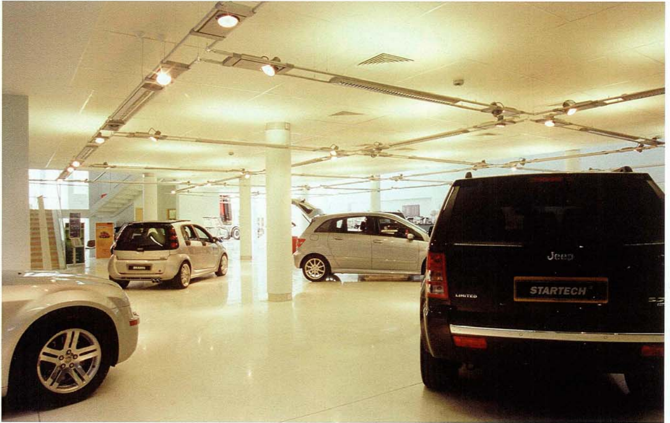
A Trilux T-200 track network was specified for the single height areas. All product sourcing and supply was provided by Storm Lighting Solutions
